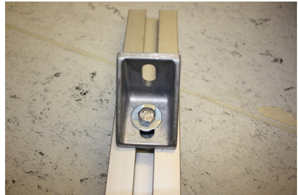
Figure 27: Bracket positioning
